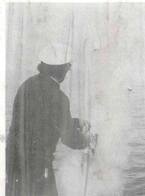
1. Firing 'Speedline' with buoyant head on rocket. Above: 'Speedline' self-contained line-throwing apparatus.
