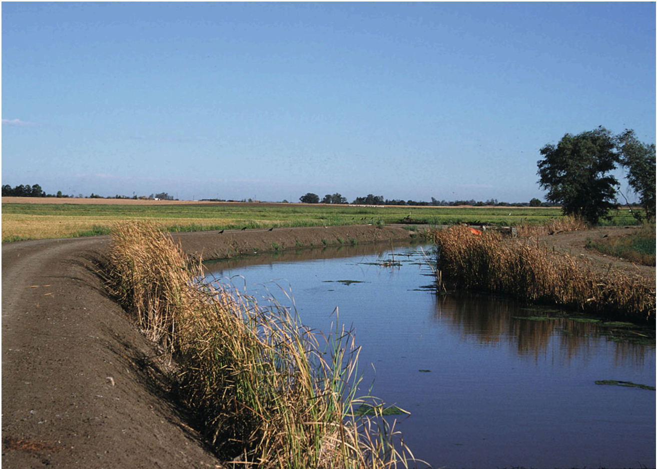
Fig. 11.7 Tailwater recovery channel (Credit NRCS Jeff Vanuga)
