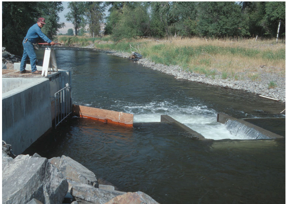
Fig. 11.4 Irrigation turnout upstream from dam in stream
