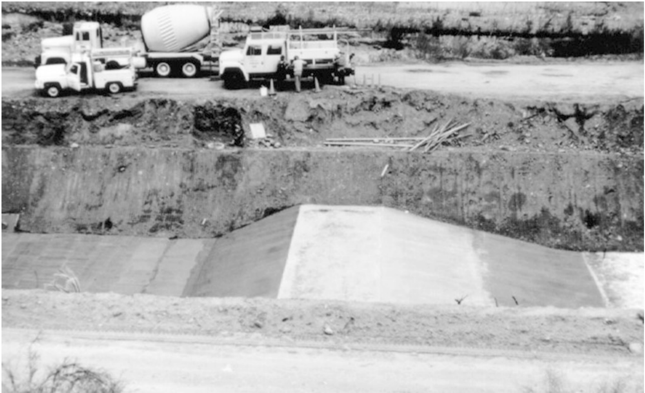
Fig. 11.26 Large long-throated flume under construction (Credit U.S. Water Conservation Laboratory, Phoenix, Arizona)
