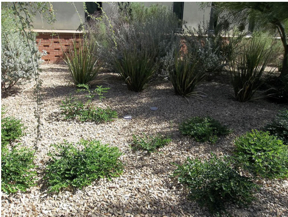
Fig. 15.5 Multioutlet emitter valve cans in landscape
