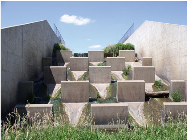
Fig. 11.16 Baffle chute energy drop structure (Wikipedia)
