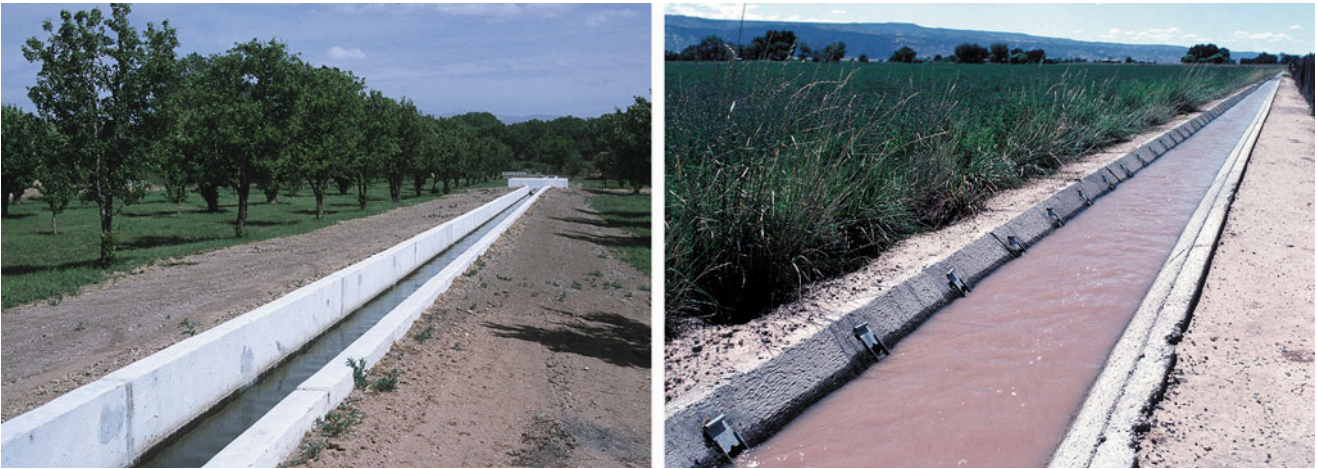
Fig. 11.1 Square and trapezoidal irrigation ditches (Credit NRCS)
