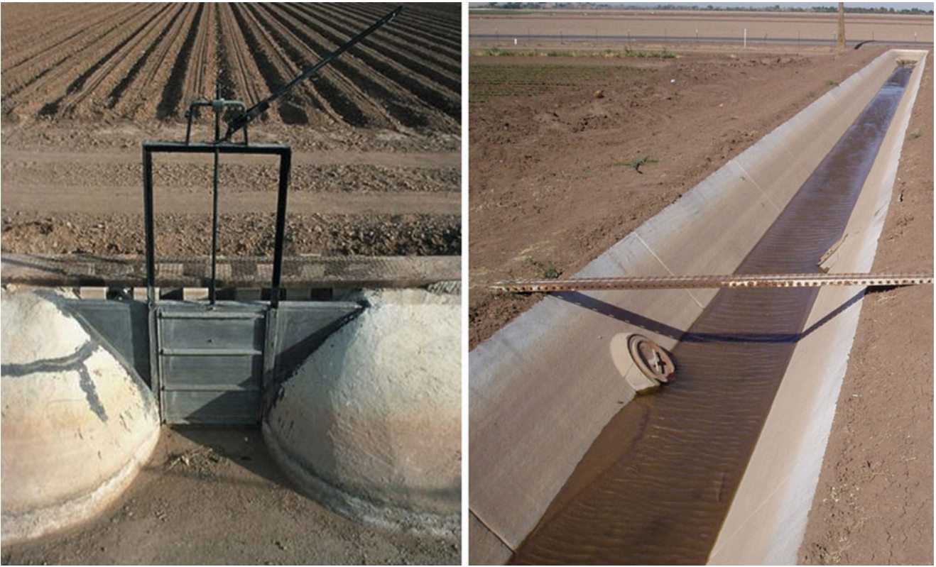
Fig. 11.5 Slide gate in farm irrigation ditch bank with energy dissipation blocks to prevent erosion ( left ) and spill ( right )
