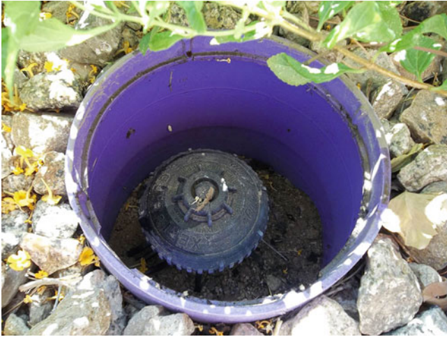
Fig. 15.4 Multioutlet emitter in valve can
