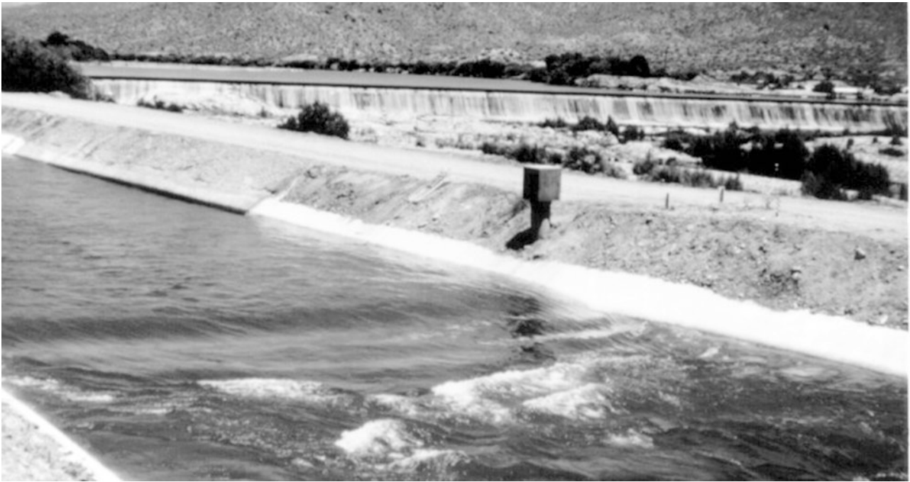
Fig. 11.27 Large long-throated flume under operation for left to right flow (Credit U.S. Water Conservation Laboratory, Phoenix, Arizona)
