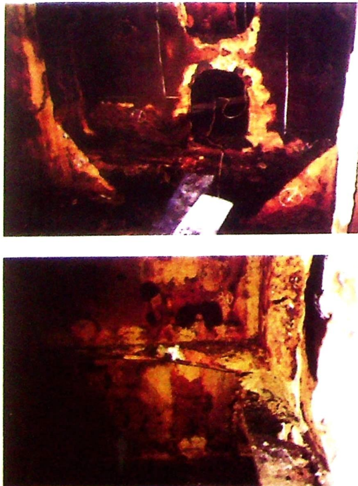
Figure 1.8: Local Corrosion in Way of Coating Failure, Coated Segregated Ballast Tank
