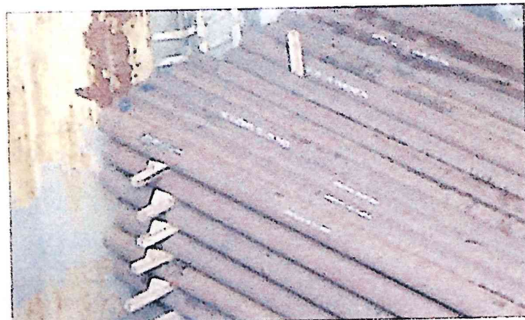
✓ Wooden wedges used to secure the pipes horizontally
