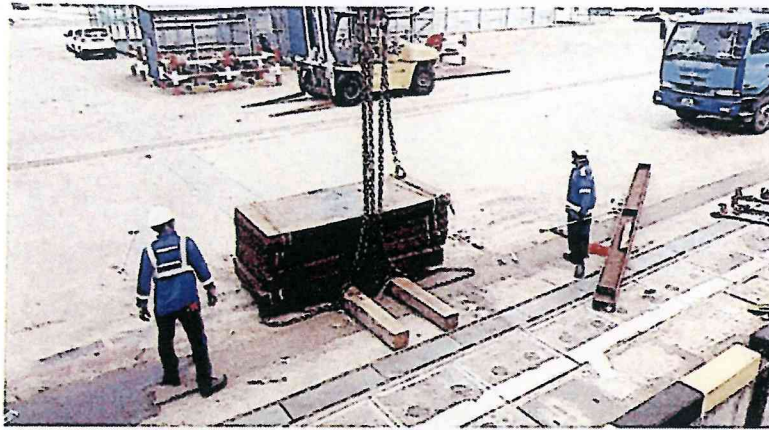
✓ Bundled, palletised, prefabricated steel plates
