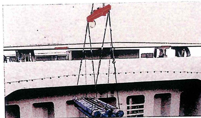
❌ Bundled pre-slung pipes being loaded by basket lift Note: the use of wire slings will damage the packaging and the pipes. Nylon slings should be used for the basket lift
