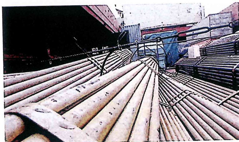
❌ Loose and badly secured pipe bundles
